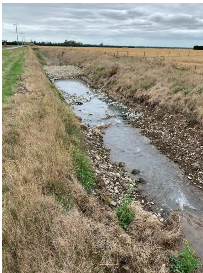
Figure 3-6: MAR 02, Timaru Track Rd. MAR lateral race (Source: B. Painter)
