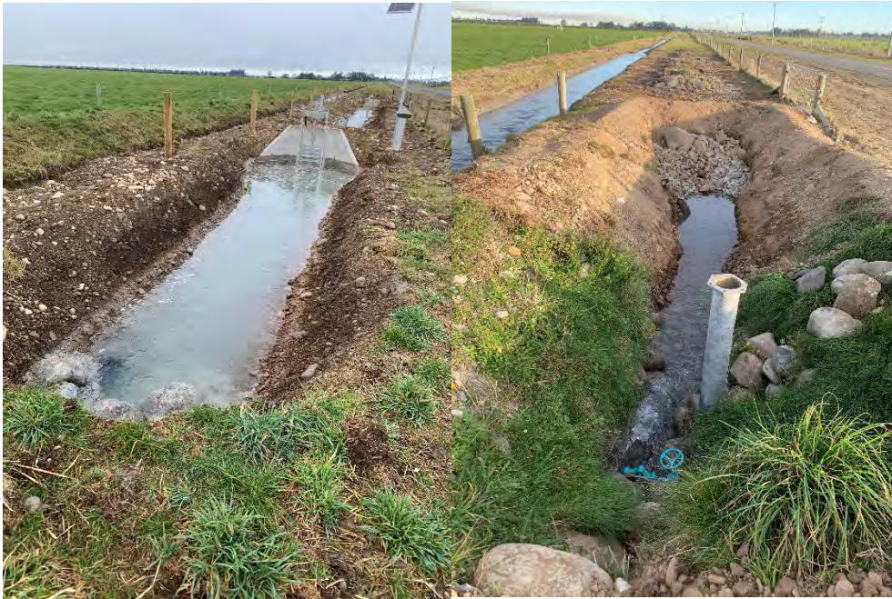
Figure 5-6: MAR 12, Maronan Ealing Road, up gradient (left) and down gradient (right)
