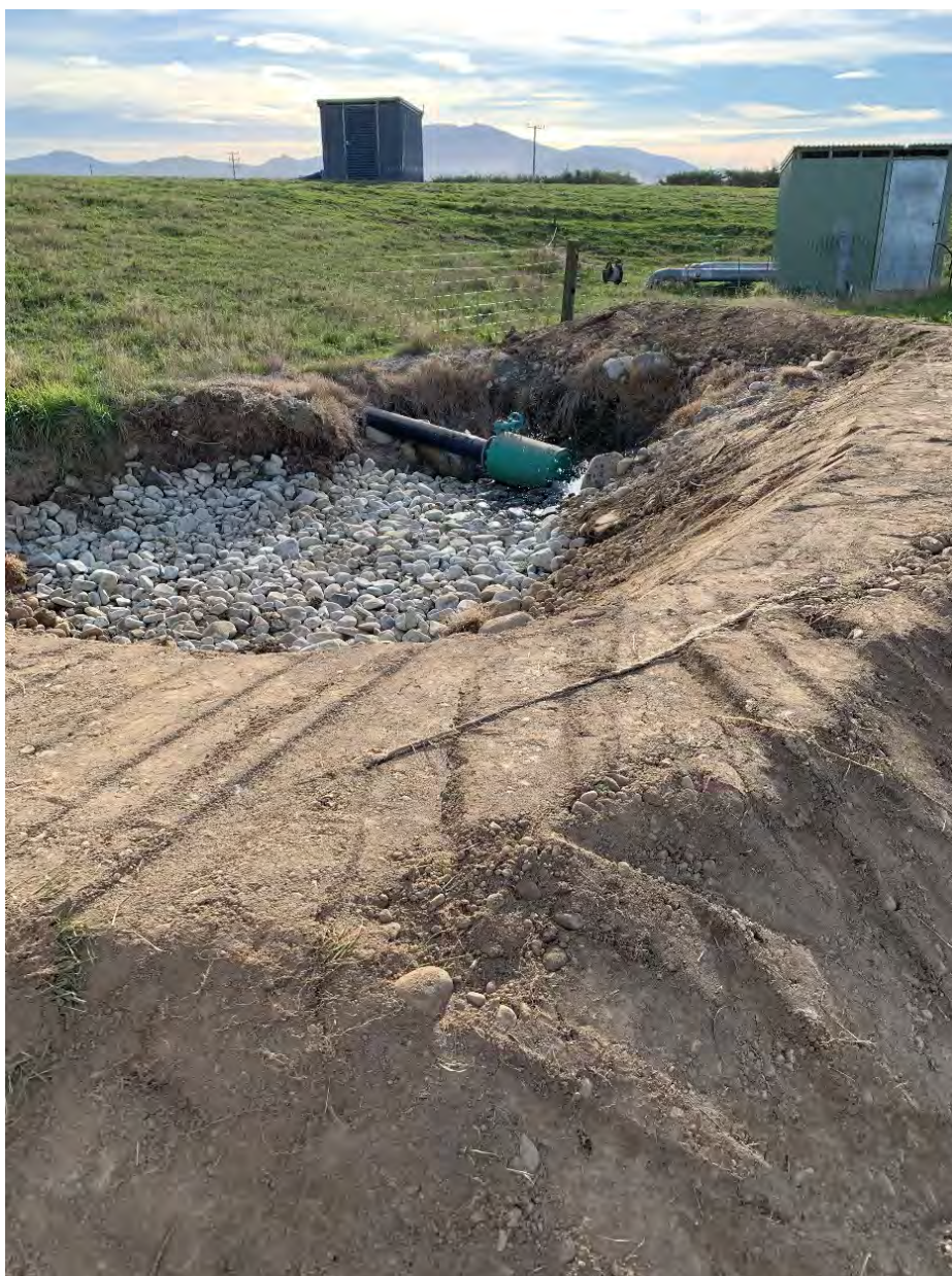
Figure 5-8: MAR 13, Hinds Arundel Road
