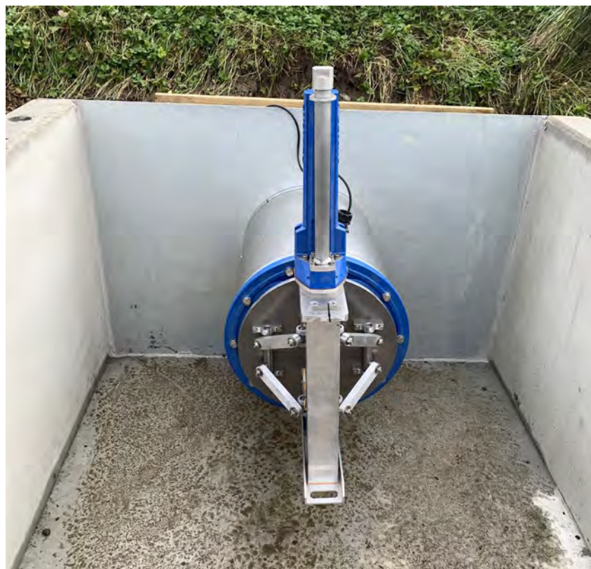
Figure 3-3: MAR09: New Rubicon 300 mm Rubicon Blademeter (Source: M. Neutze)
