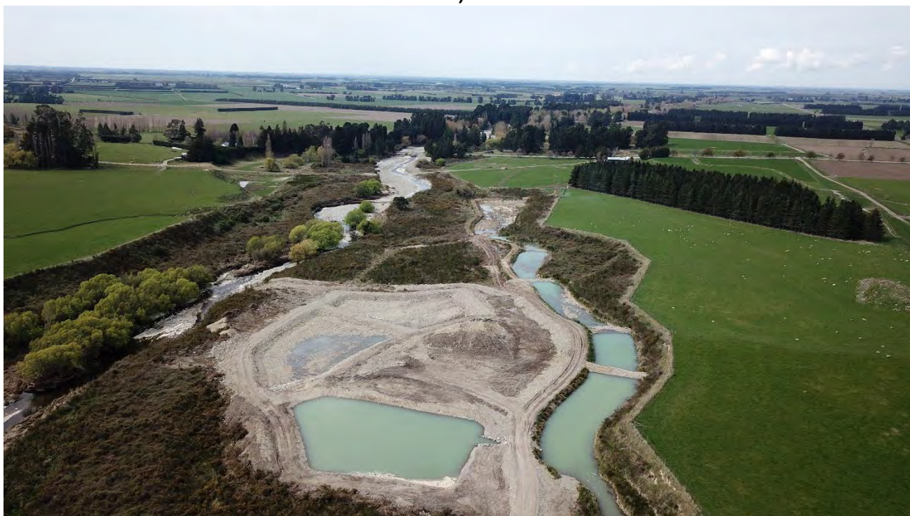
Figure 2-4: NRR1 site original (right) & new (left) recharge basins, October 2021 (Source: HHWET)
