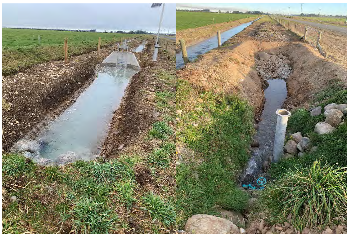
Figure 3-3: MAR 12, Maronan Ealing Road, up gradient (left) and down gradient (right). MAR test site enhanced with buried slotted pipe (Source: M. Neutze)
